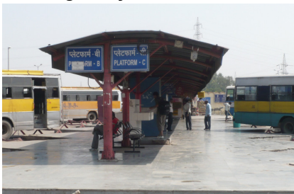
Platform and Passenger Shelter
