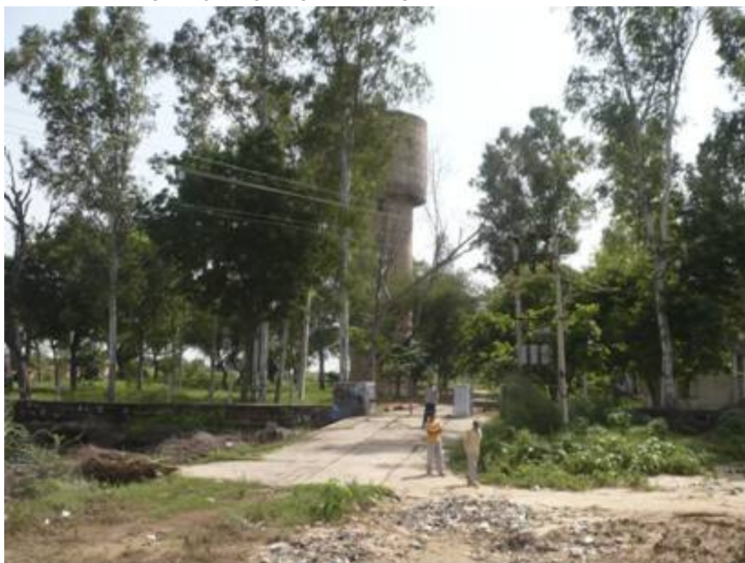
FIGURE 1.2 : ELEVATED SERVICE RESERVOIR IN PATAUDI
